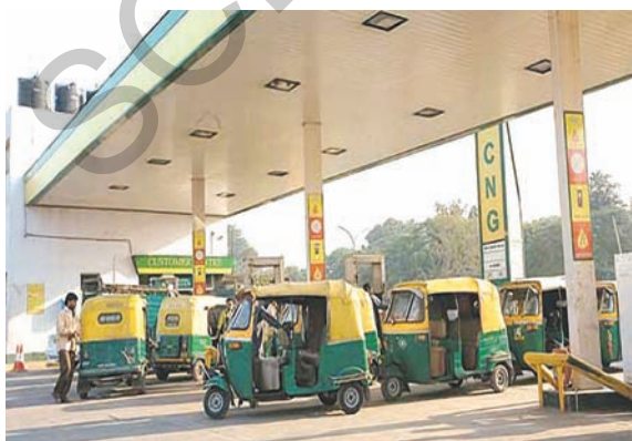
Fig - 3: CNG filling station
